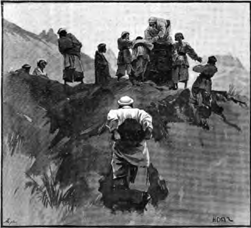
BUILDING A STONE-MAN AT BOGGY CAMP.
